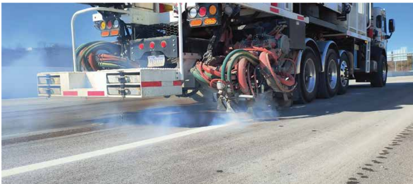
Thermoplastic pavement marking on an interstate highway by A&A Safety.
