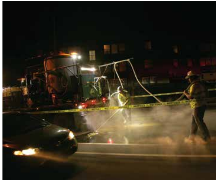
A&A Safety crew installing high-friction surface.
