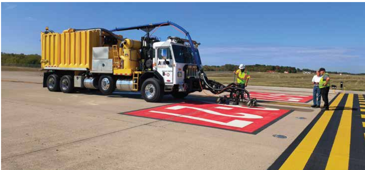
A&A Safety truck removing old runway markings before new markings are applied.
